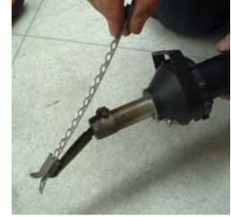
3. Firmly weld the stripe into the groove. Proceed in small steps, in stop-and-go manner, each time applying adequate pressure on the repair nozzle. When completed, firmly pull on the stripe to test the welding result. If the stripe comes off easily, start over and set a higher temperature.
