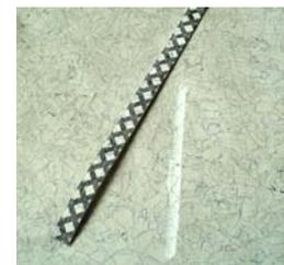
2. Set the welding gun temperature to approx. 450° C / 840° F. Slide the stripe into the flat repair nozzle, bottom side up. Prior to proceed, test the temperature on the Colorex stripe. The material should just become very soft, however without melting down or turning brown.
