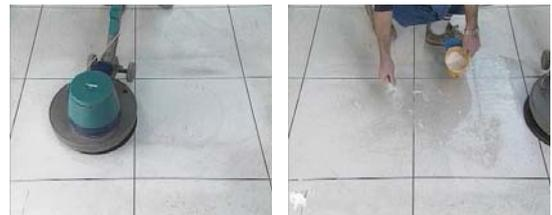
2. Remove the dirty cleaning solution with a wet vac. Rinse with clear water to remove abrasion dust and wet vac as well. At this point, the floor will be visually clean but the surface will be quite rough and needing to be restored.
