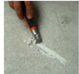
5. When cool, trim the welding flush with the floor using the eccentric grinder. Start with a coarse sandpaper grade (120) and proceed in several steps up to 240.
