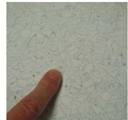
6. Complete by restoring the original surface smoothness of the repaired and grinded spot by dry polishing with a blue pad first and then with a red one. You can skip this passage if a restorative maintenance is to follow.
