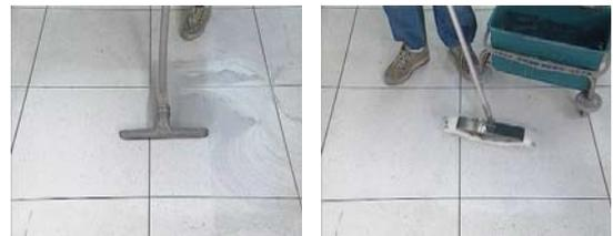
3. Restore the original surface smoothness and quality by dry polishing with the low speed single disc machine and pads in decreasing degree of abrasiveness. Start with the green or blue pad and then continue with the red one. If a shiny appearance is required, dry buff with the yellow or white pad.
