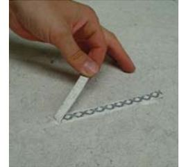
4. While still warm, remove excessive parts of the stripe with the crescent shape knife and/or sharp scraper and then allow the repair to cool down completely.
