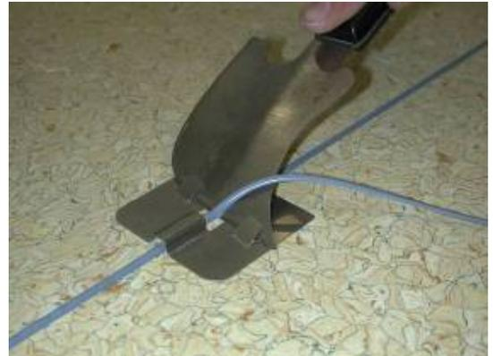
4. For the second phase, wait until the remaining excess is cold, then trim flush using a sharp crescent-shape knife. Tip: use a separate, clean and extremely sharp knife dedicated to that purpose.
