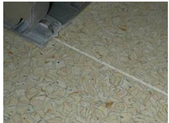
2. Weld the Colorex welding rod into the clean groove by means of the automatic seam welding machine. Use the hot air welding gun and quick welding nozzle for difficult to reach areas. Welding temperature to be 400° - 450°C.
