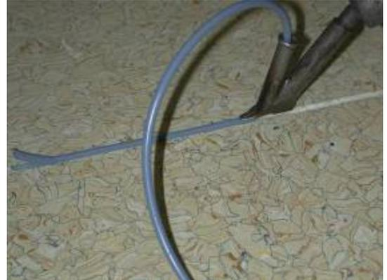
3. It is highly recommended that trimming is done in two phases. In the first phase, while the welding rod is still warm, trim off part of the excess welding rod with the crescent-shape knife and the trimming slide.
