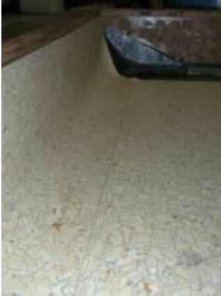
Skirting cut flush with floor tiles.
