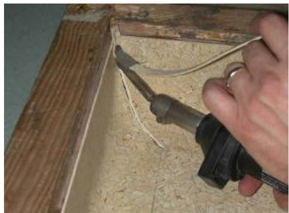
...weld the stripe firmly into the groove, starting from top
