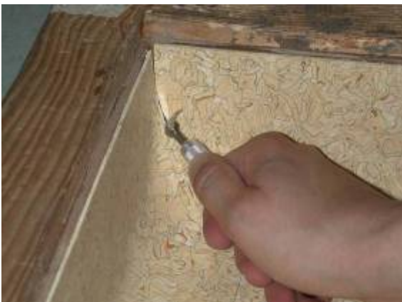
Next, groove skirting junction lines in corners,
