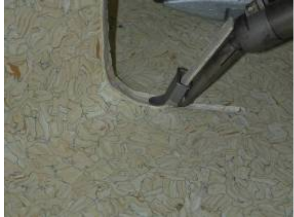
Afterwards, weld the remaining part with the flat welding nozzle
