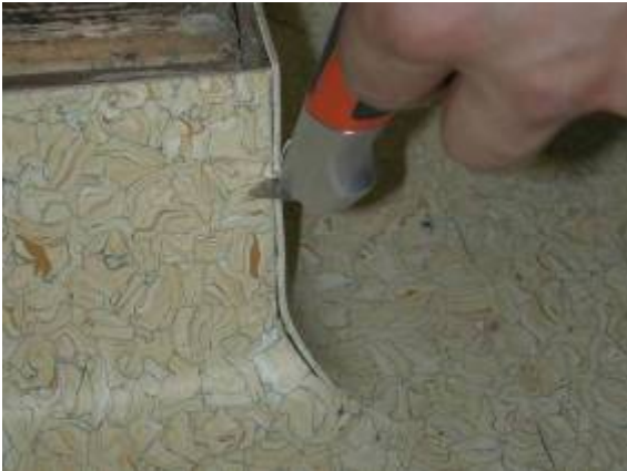
Angles must be grooved too, as shown
