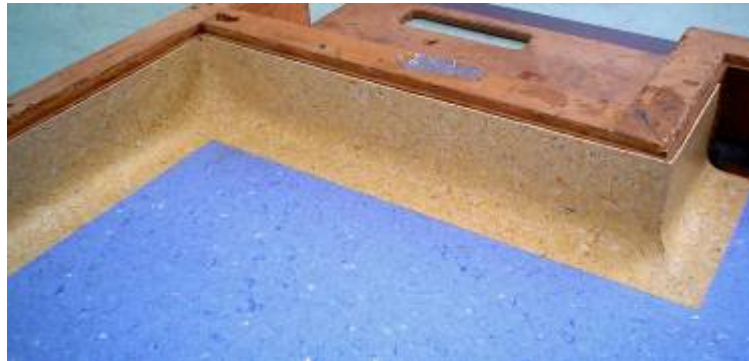
Seam welding missing for illustration purposes
