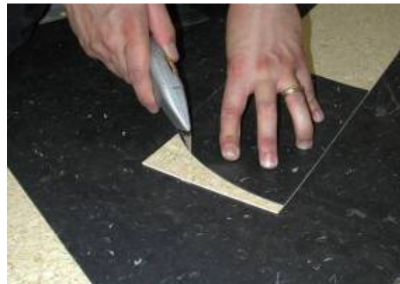
Scarify the skirting end using your template...
