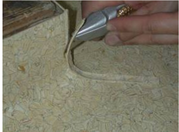
Cut excess material with knife...
