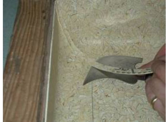
While still warm, remove excess material with a sharp crescent shape knife.
