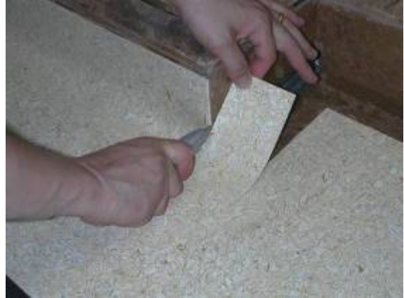
Continue with skirting application. Cut outer corners as shown.
