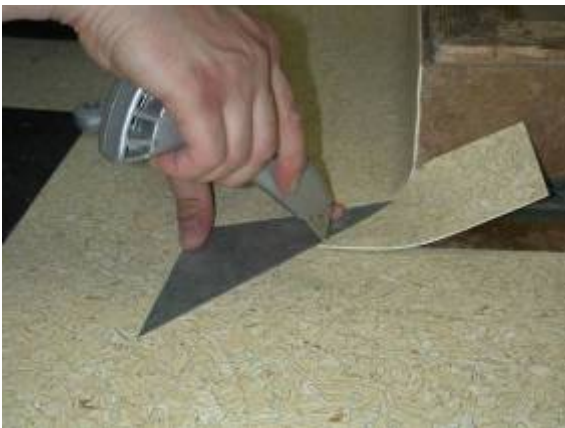
Always use a metal guide for these operations
