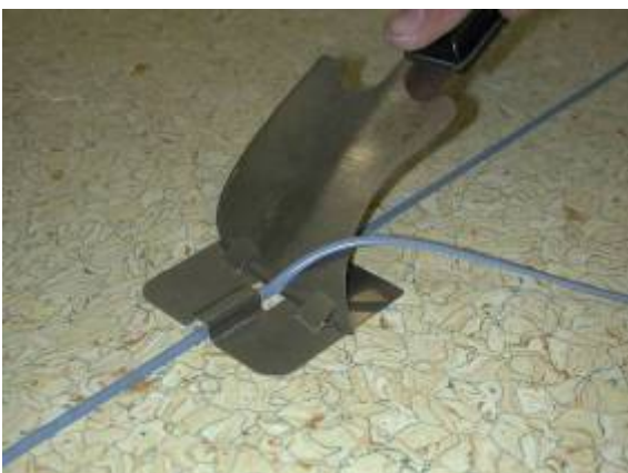
1 st passage: trim with slider and knife while still warm
