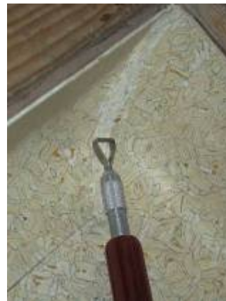
Use round or triangle hand grooving tools as needed
