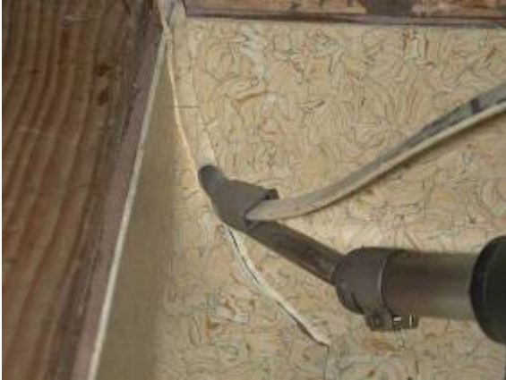
Set welding temperature to approx. 350° C, adjust if necessary
