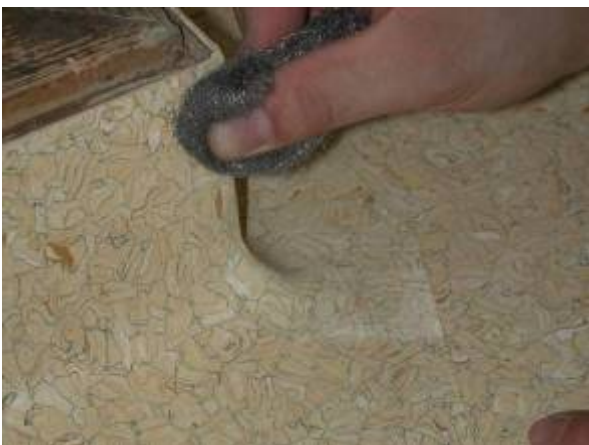
...you can finish off the weldings
