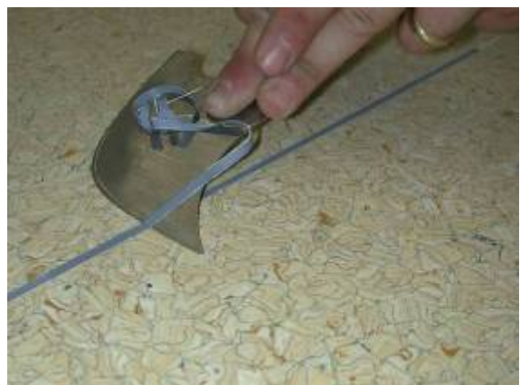
2 nd passage: when cold, flush trim with sharp crescent shape knife.
