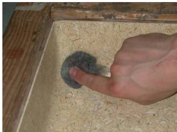
Acetone will make the sanding traces disappear.
