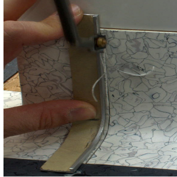
Groove the joint
