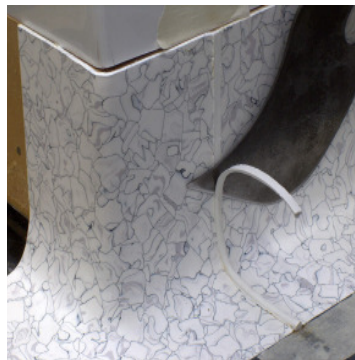
Once applied roughly remove the excessive weld.
