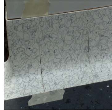
Protect the parts that don't need welding with adhesive tape.
