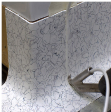
Weld with appropriate PVC weld ( hot air 300/350 °C)
